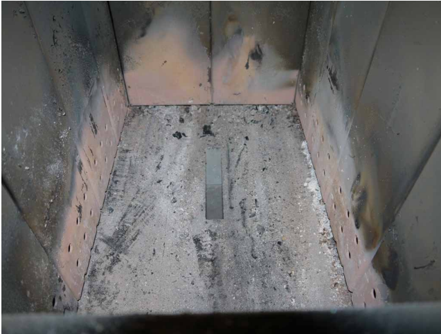
Figure 6 Correctly cleaned feeding chamber
